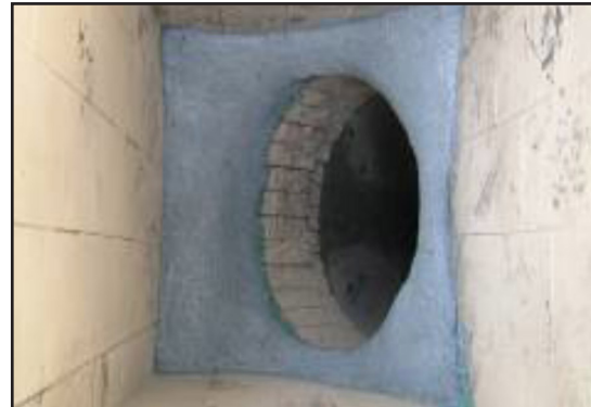
Installation of ARC BX5
