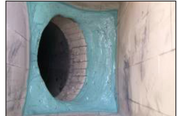
ARC BX5 with ARC S2 topcoat cures rapidly, allowing fast return to service of chute
